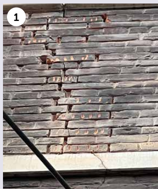
Above left to right: 1. Identifying the scope of brick stitching; 2. Insertion of helical fixing bars and mesh; 3. Replacement bricks; 4. Disguising the repairs with staining
